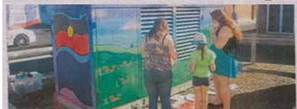
ANZAC PROJECT: Members of Casino Youth Early Intervention Service, Chloe, Lili and Stephanie do the stencilling of their Anzac Public Art project thanks to funding by Richmond Valley Council and support by Essential Energy who allowed their substations to undergo the make-over. Co-ordinator Annika Olsson said the murals were a way to recognise the contribution of the many Aboriginal and Torres Strait Islander people in international conflict since the First World War.
